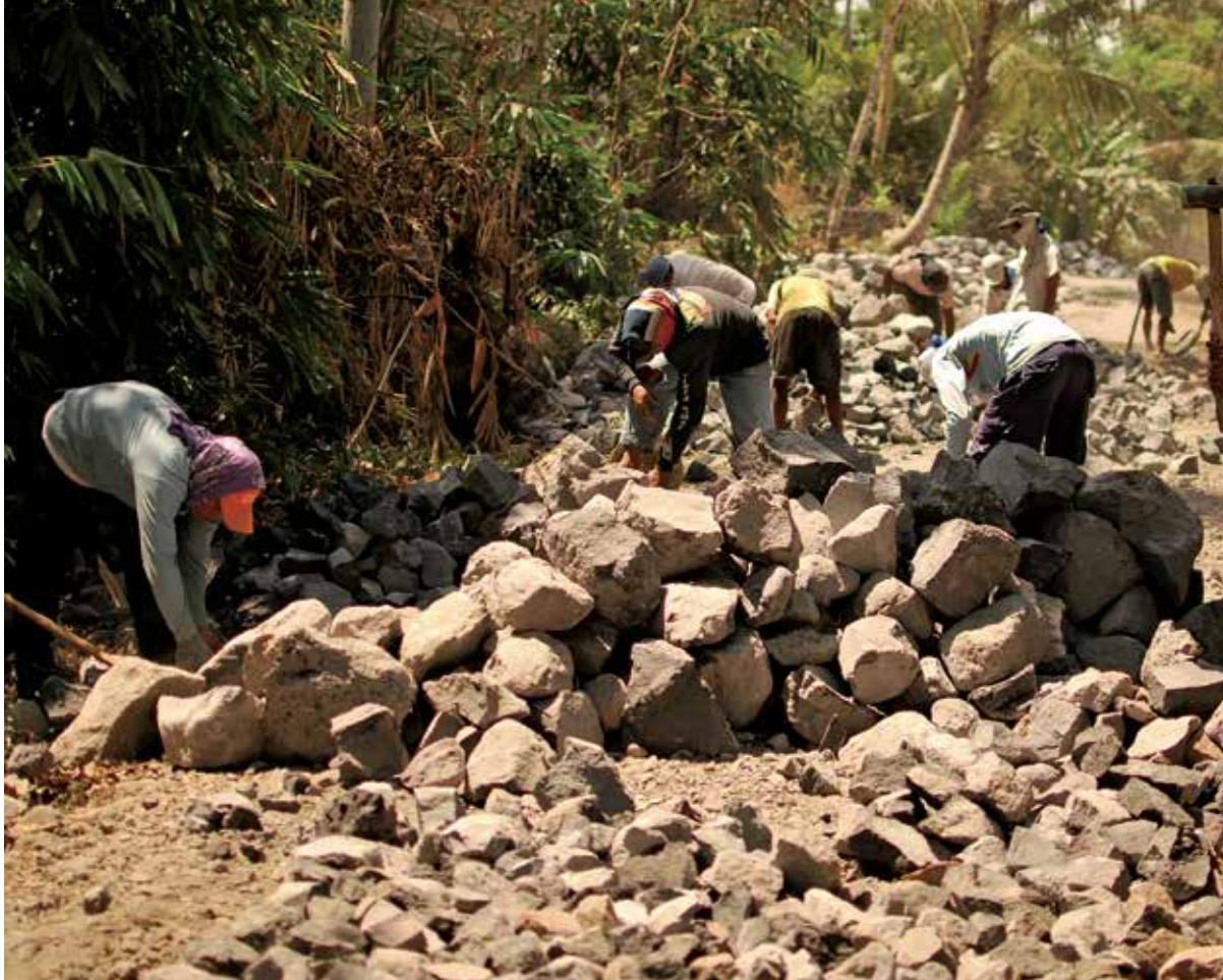
Rebuilding a road after eruption of Mount Merapi in Yogyakarta, Indonesia (World Bank).
