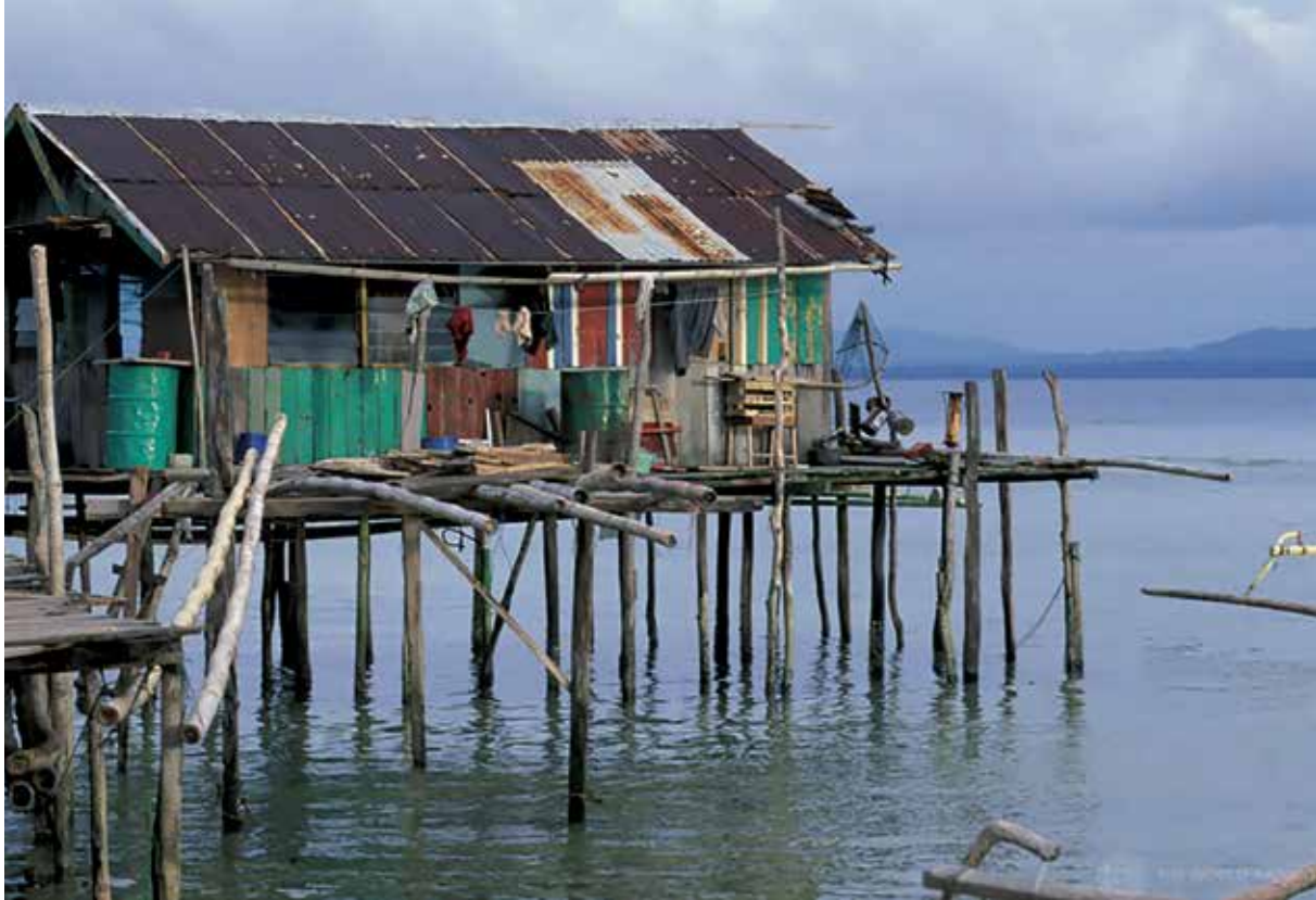
A house in Indonesia built on stilts to protect against flooding (World Bank).
